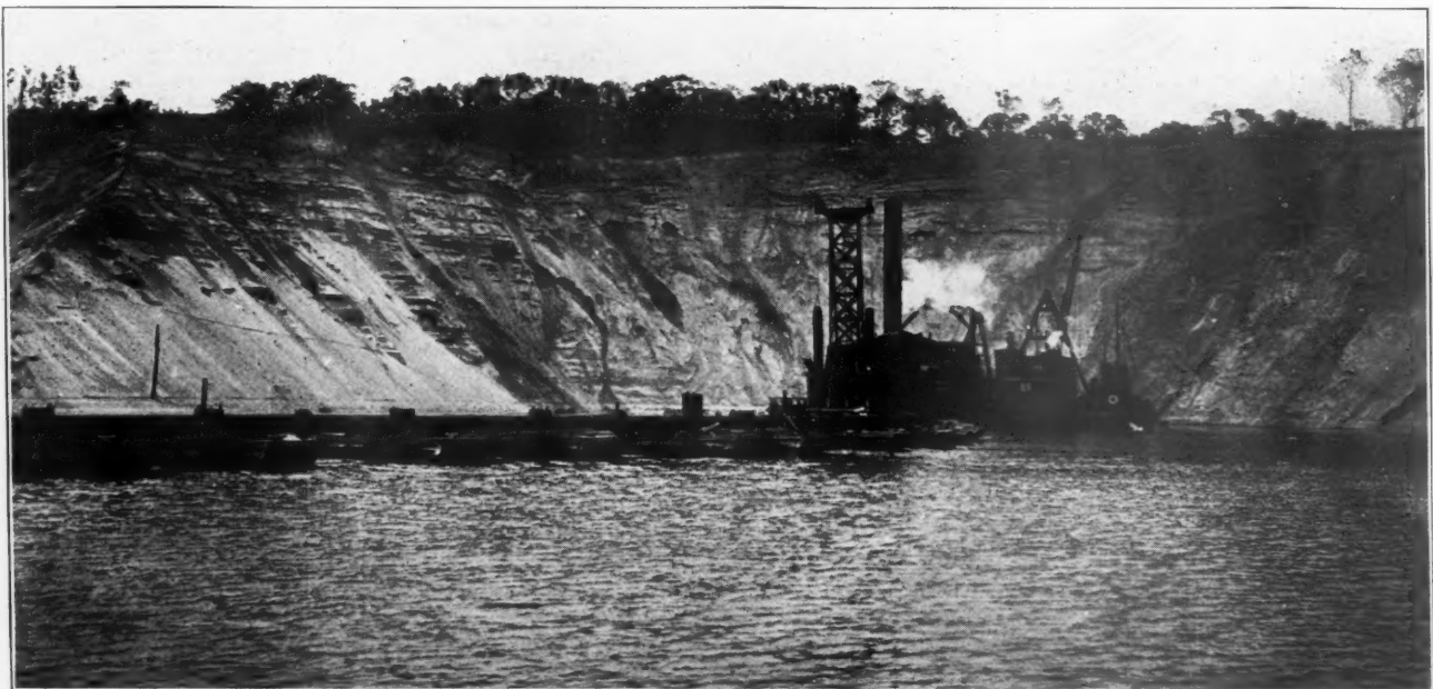
Dredge and Pipe Line Supported on Pontoons. Note Height of Bank
